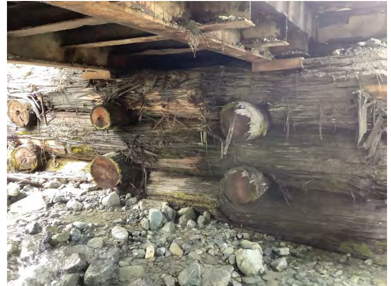
Left Bank Abutment when facing downstream
