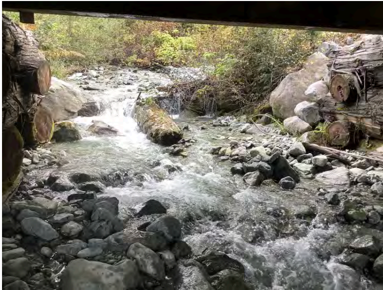
Upstream from Crossing
