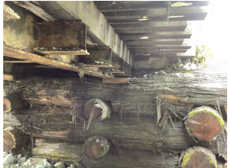
Left Bank Abutment when facing downstream
